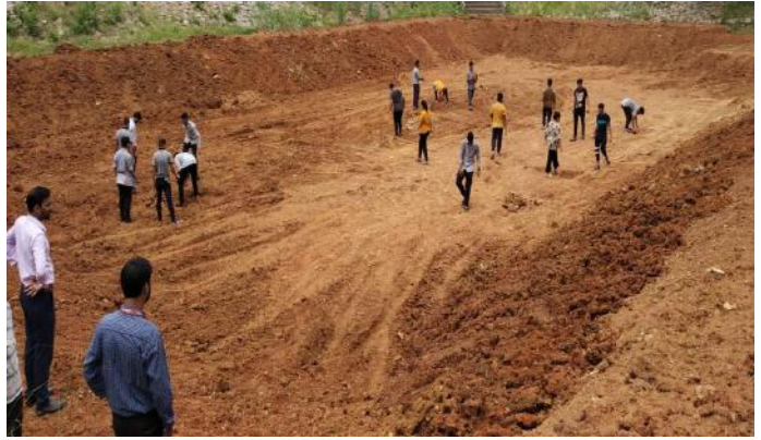
PREPARATION OF POND FOR LINING
