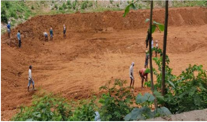
PREPARATION OF POND FOR LINING
